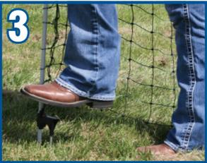
When installing the post, the step-in part of the post should be placed at a 90° angle to the net. Once all posts are installed, tie the first post to the last post with the green strings.
