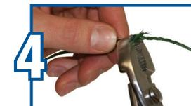
With a pair of pliers, crimp one end of the sleeve over both pieces of twine.
